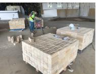
processes of cleaning the 5,000 bricks that will be reused (left) in the new entryways and rooms. Front e n t r y
